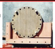
2 Gaskets are placed in position and the top saddle section is bolted into position.
